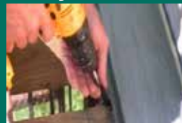
Screw to Joists
