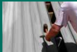
Lay Down Deck Board
